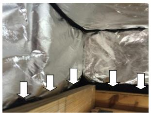
Put a bead of silicone sealant along the gaps as close as you can to the stapled foot.
