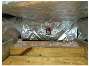
Adjust the Velcro straps on the outside of the ThermoClimb to fit snugly against and around the frame. Use a stapler to staple flat the cover to keep air from escaping.
